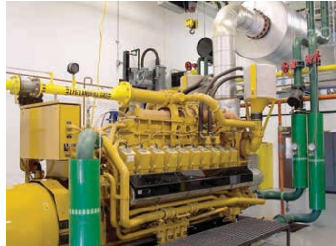
project reasonably assumed that there were significant 3rd harmonic generating loads in the system and that each generator would need its own neutral harmonic filter.
